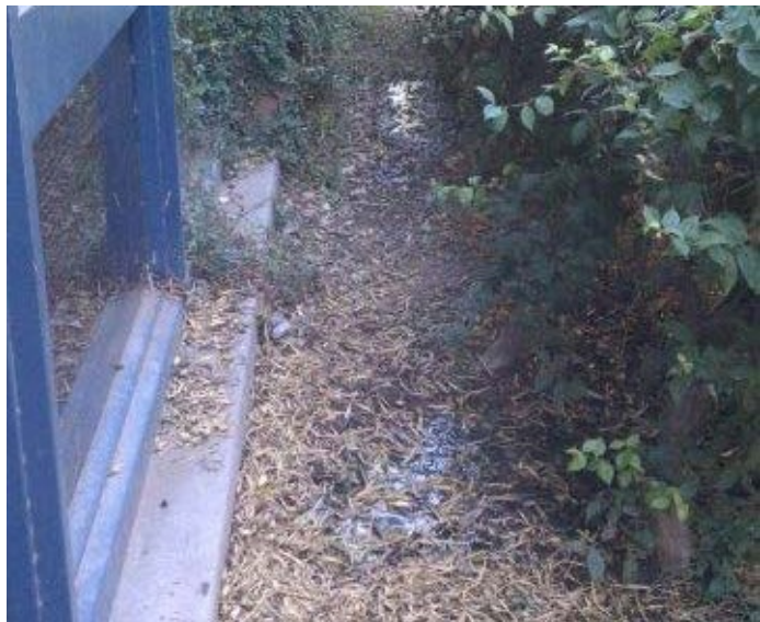
Fig. 6. Fallen leaves and other debris around the building provides harborage for pests and also holds moisture which can weaken the foundation.
