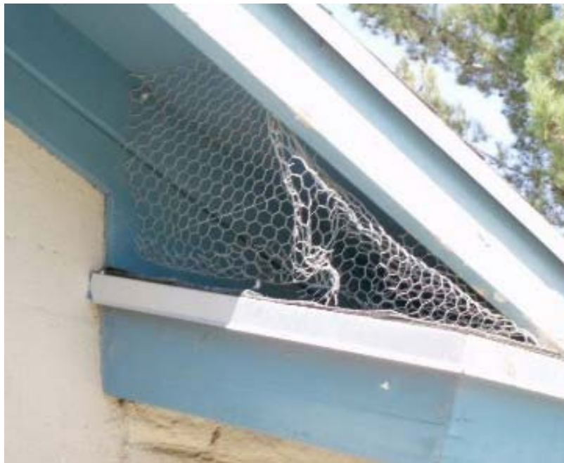
Fig. 7. Wire netting helps to keep birds and rodents out, but needs to be monitored and maintained.
