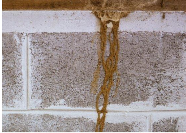
Subterranean termite-working tubes Photo: USDA-Forest Service
