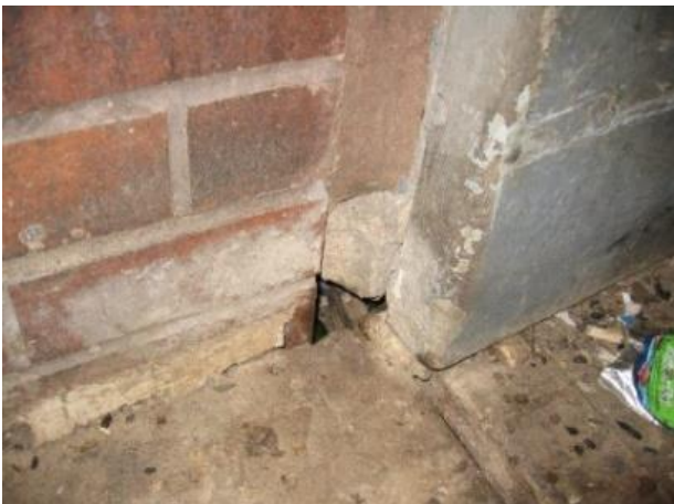
Gaps or holes in walls or foundations provide entryways to rats. Photo: Dawn Gouge
