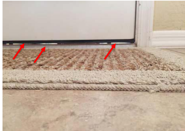
This locked door is wide open to pests! See light coming in through gaps under door.
