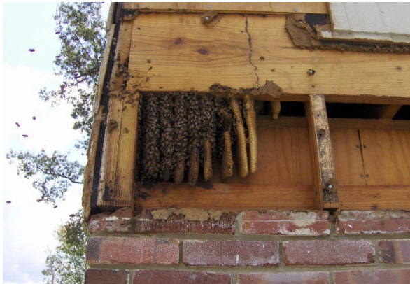
Figure 5. Honey bees established inside the siding of a home, after entering through a crack in the wall. Photo: Timothy Haley, USDA Forest Service.
