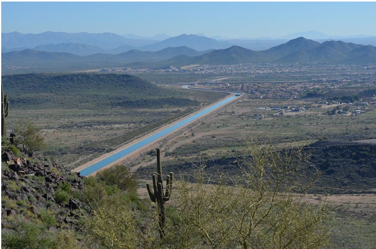
Figure 1: Central Arizona Project Canal in Phoenix, AZ in 2010. (Photo: User: Onel5969, Wikimedia Commons)
