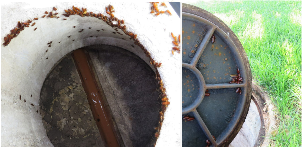
Figure 5: American cockroaches inside a sewer and a manhole lid. (Photos: Dawn H. Gouge)
