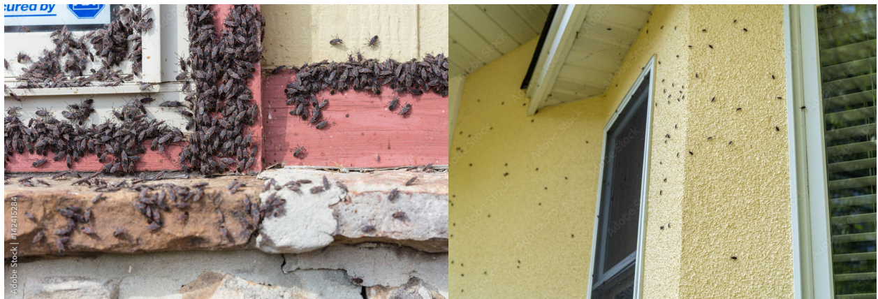
Figure 2: Aggregations of bugs, left - outside a home entrance (Photo: Melinda Fawver), and right - on exterior walls (Photo: Melissa MN).
