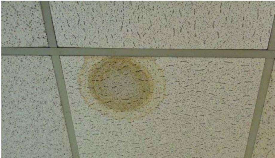
Figure 5. Ceiling tiles indicating a roof or plumbing leak.
