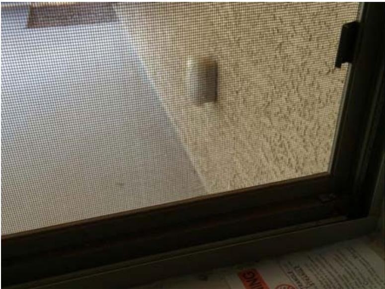
Fig. 7. Screens (18 x 18 mesh) on windows and doors help to keep out most flying insects.
