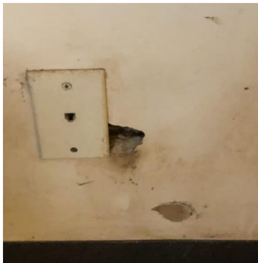
Figure 9. Rub marks confirm rodents are entering the gap next to the faceplate. Photo: Susannah Reese, StopPests
