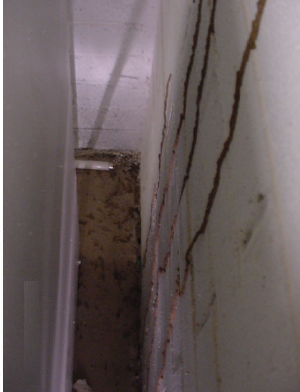
Figure 9. Subterranean termite shelter tubes on a wall behind a piece of equipment. Photo: Dawn H. Gouge
