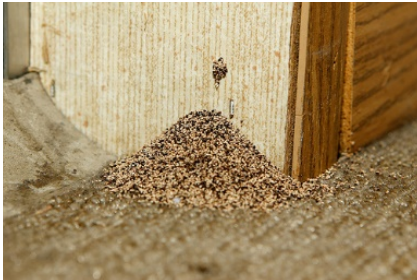
Figure 11. A pile of drywood termite fecal pellets below a bore hole.
