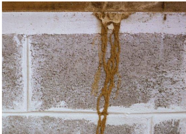
Fig. 8. Subterranean termite shelter tubes. Photo: USDA Forest Service
