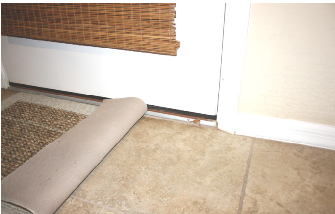
Figure 9. The scorpion likely entered through a gap in the weather-stripping around the door
